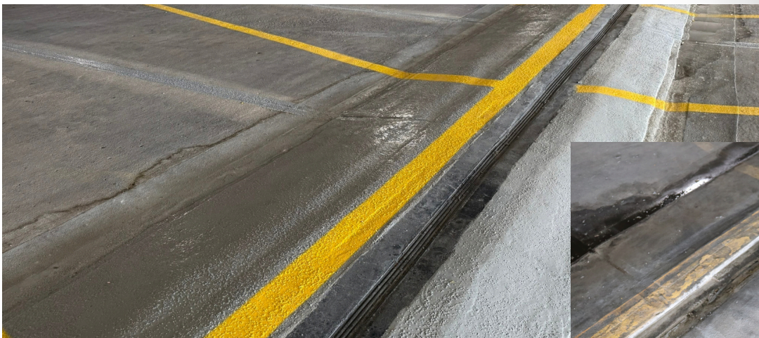
Completed installation of Nystrom Seismic Wing Parking System, restoring long-term performance.
