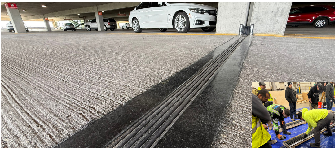
MSP completed expansion joint installation.
